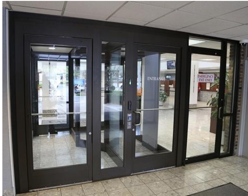
Picture 40 – Man Trap Doors - Standard Telephones and Cables
