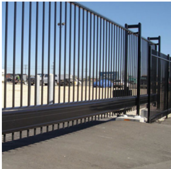
Picture 8 – The Delta Cantilever Sliding Gate
